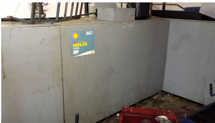
A contained room of bulk oil. The tanks are also double skinned.
